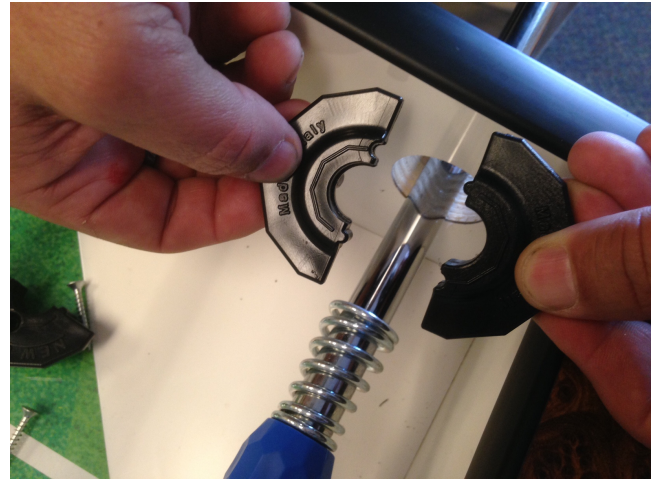
From the playing surface side, pair two of the positive and negative part that have NO screw holes and push them against the rod and into the opening
